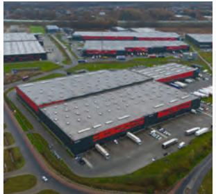
KOKOTÓW - Main warehouse
